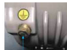
earthing connection terminal
