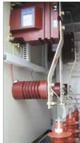
internal view of service compartment for line units
